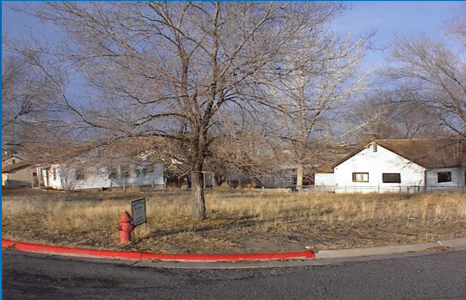
Abandoned Residential Lot
